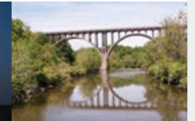
View of Route 82 bridge from towpath, Cuyahoga Valley National Park
