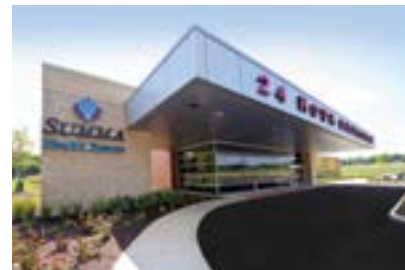
Summa Health Center Emergency Department at Green 1825 Franks Parkway, Uniontown, OH 44685
