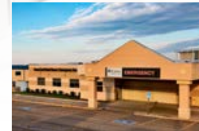
Summa Health Center Emergency Department at Wadsworth-Rittman 195 Wadsworth Rd., Wadsworth, OH 44281
